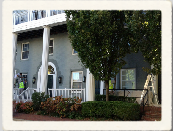
Building 2 Gets a Fresh Coat of Paint
