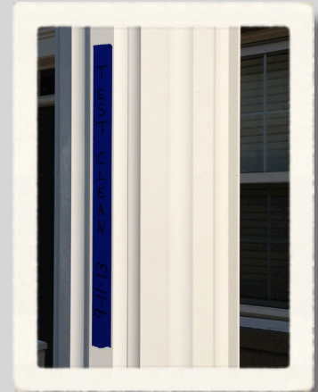
A Column After Cleaning
